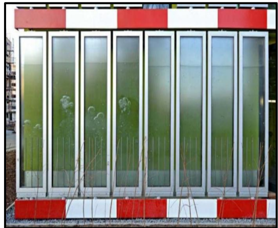
Glass panels filled with liquid biomass material (algae) that are able to supply its own electricity.
